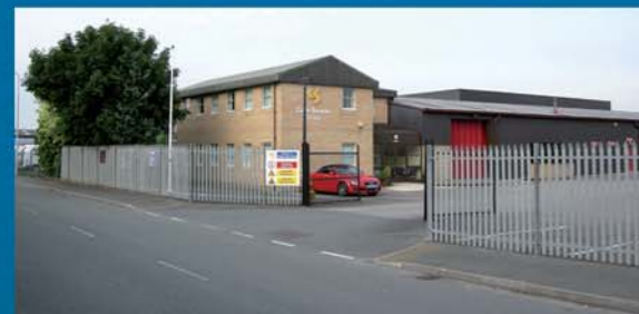
Cable Services International Offices
