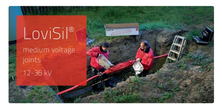
LoviSil<sup>®</sup> medium voltage cable joints have been developed featuring fluid silicones that can boast 30 years proven field experience with an extremely low failure rate. Thanks to the construction and characteristics of the silicone based insulation material, LoviSil<sup>®</sup> joints offer a reliable connection with polymeric and especially paper-insulated cables.
