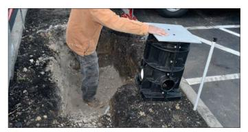
Prepare the site with subtrate dug out to accommodate a hand tamper or vibrating plate to be used on all sides of the foundation. Depth should be the height of the foundation (25") plus a 6" gravel base. Minimum gravel base: 6" or enough to reach the region's frost line.
