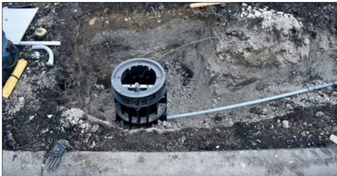
Ground prepared for installation of foundation; conduit ran and routed through open port to middle bar.
