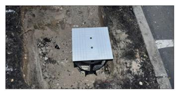
Gravel filled in, in 3" - 6" increments, and then hand- or machine-tamped.
