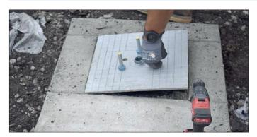
Attach the mounting bracket or plate for the charger/charger stand. Suggested use is to put star lock washers on to hold the bolts in place as the lid is bolted back down to the foundation.
