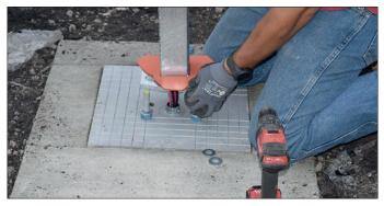
Once holes are drilled, bolts are mounted, and wire has been run, secure the plate down using the two M12 bolts. Clean the outer edges for a secure fit.
