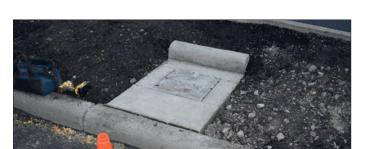
A charging-ready street showing a future proofed, scalable, pre-prepared PLP EV charger foundation. EV chargers can now be installed without any further infrastructure interruption. You may finish with concrete, paving stones, grass, mulch, or gravel.
